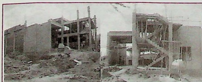
Lanka Salt Ltd, Hambantota, Progress of Civil Work
