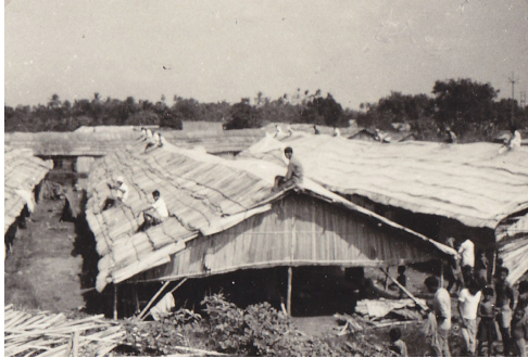
Providing mats and thatch to build new accommodation ( mat brothers)
