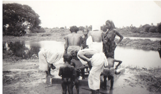
River water and borewell with pumps – the only source of water
