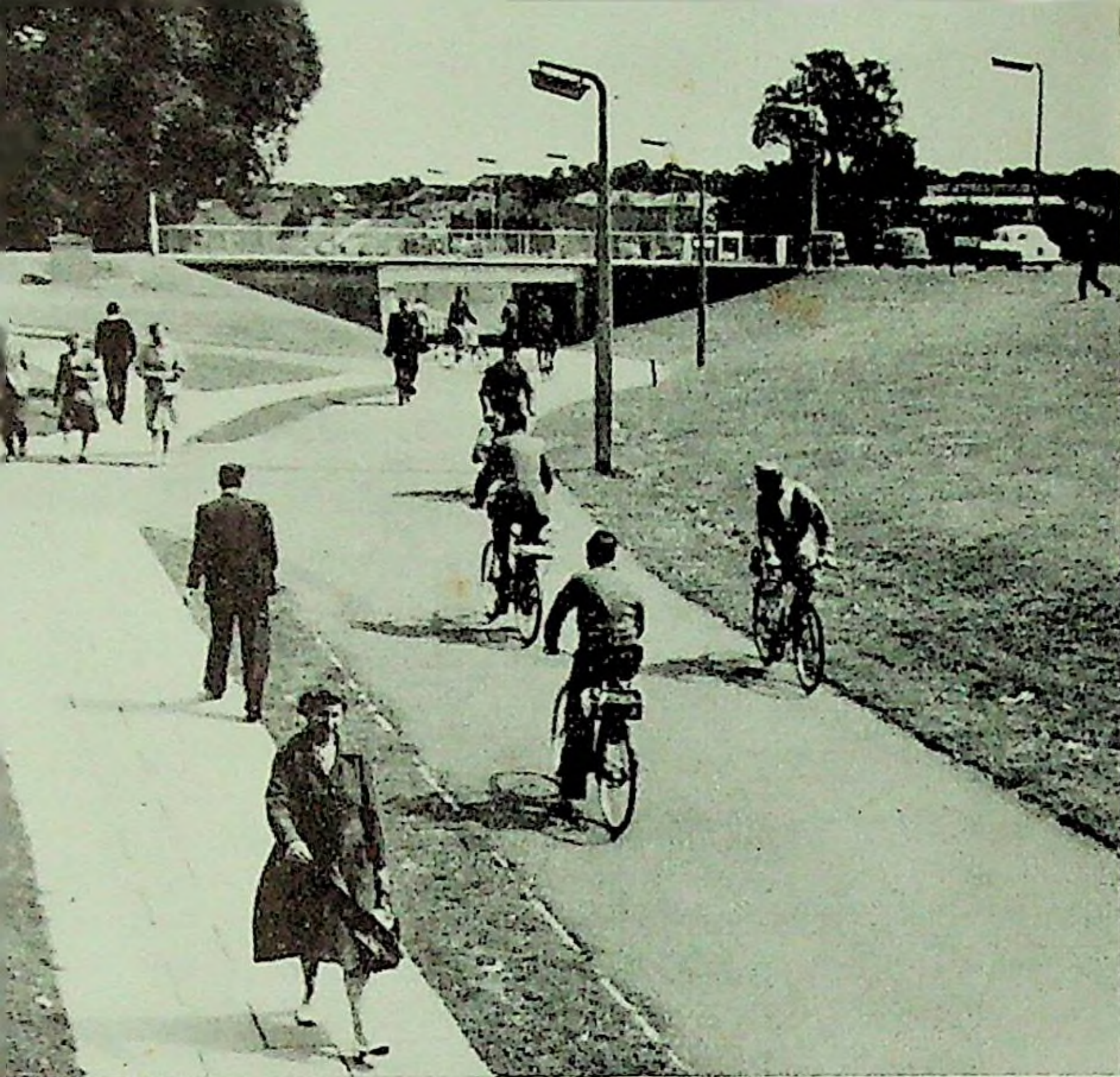
Segregated cycle- and pedestrian-ways linking Town Centre and residential and industrial areas and underpassing main-road junctions.
