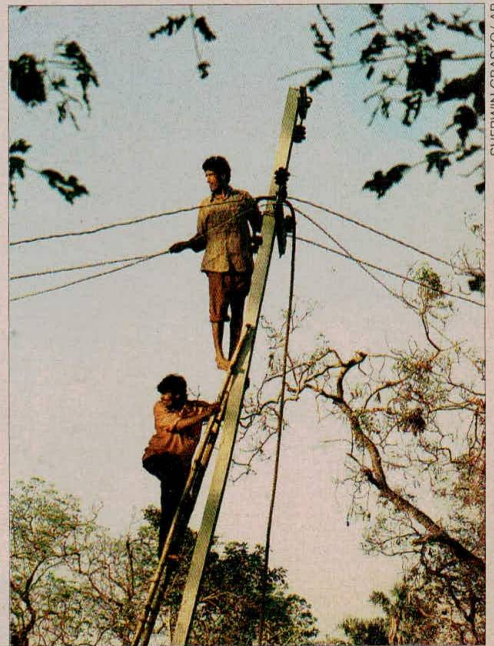
Linesmen repair power cables in Jagatsinghpur, two weeks after the cyclone.
