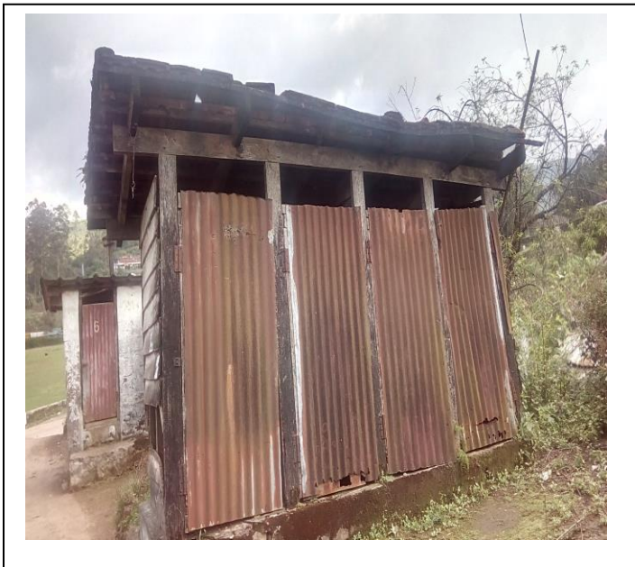
Toilets provided by the company
