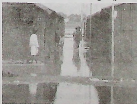
Tsunami temporary shelter in Kannagi Nagar, Chennai
