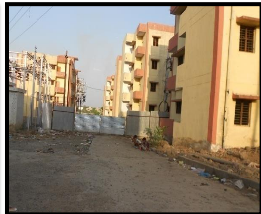
No proper sanitation, used open defecation
