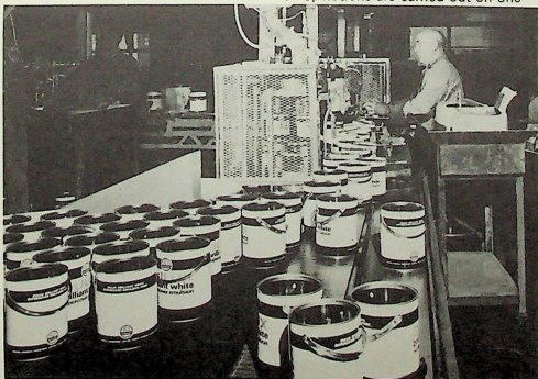
Below: Speed and accuracy are essential in filling 'Dulux' into millions of cans of different sizes. Paints Division engineers have designed ingenious machines to do the job.
