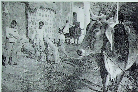
Rajokri Project Construction of Model Drain
