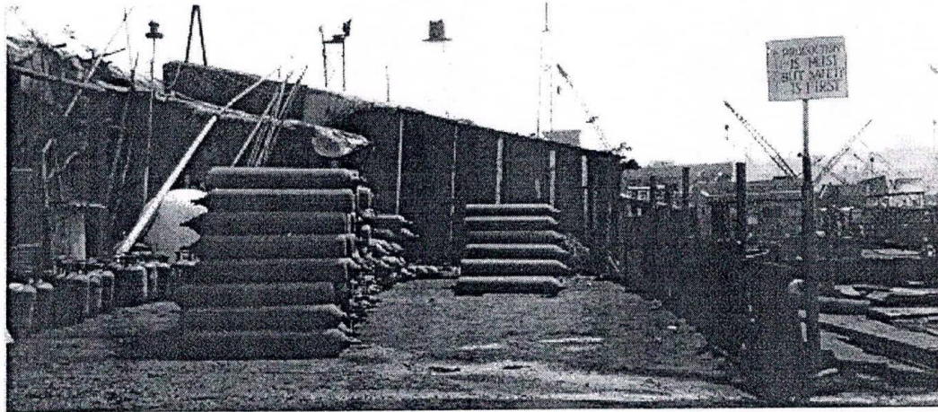
Oxygen and acetylene bottles stacked horizontally (Photo: Judit Kanthak)
