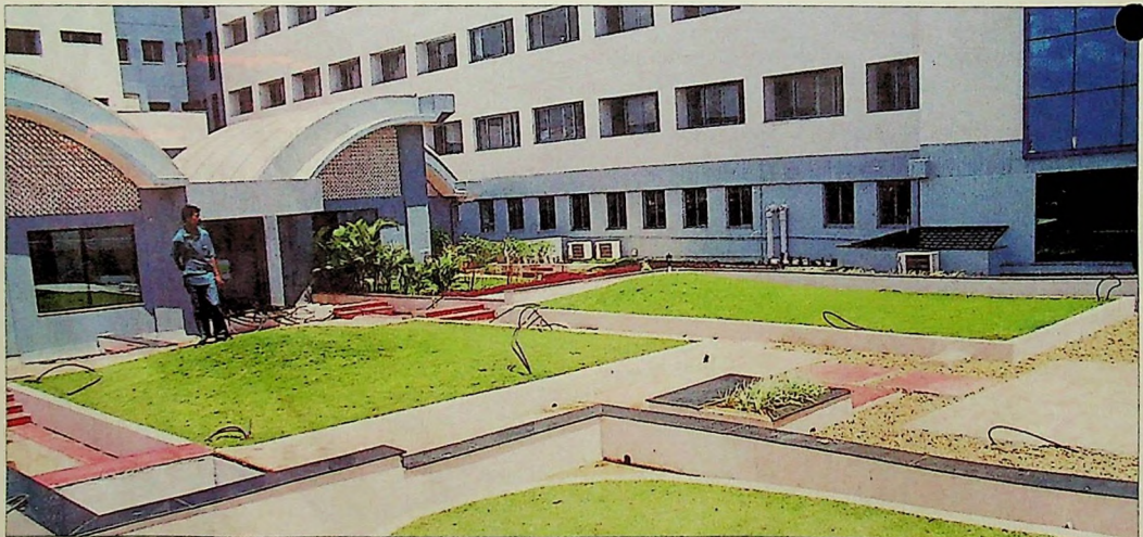
The rooftop garden for the use of inpatients recovering from surgery at the M.S. Ramaiah Memorial Hospital.
