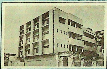
Higher course school building
