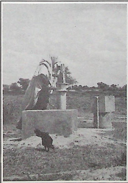
A handpump with a special storage tank in Rajasthan
