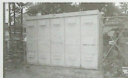
Ring Main Unit before refurbishing
