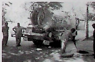
Sewer Jetting machine clearing a manhole
