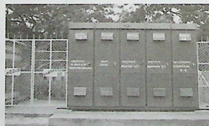
Ring Main Unit after refurbishing
