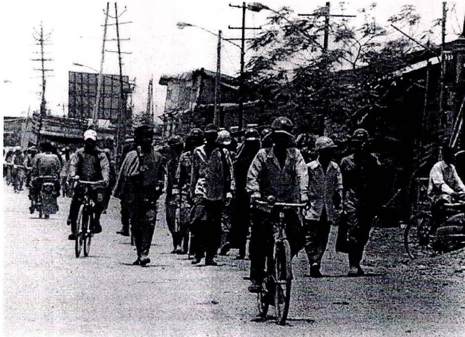
Workers using hard-hats(Photo: Santosh Bane)
