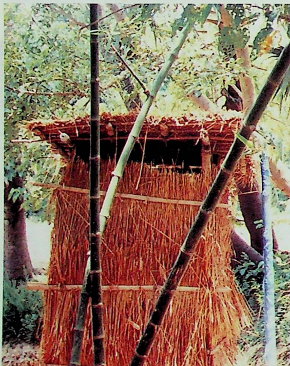
A simple but proper latrine in santal village, by the side is the gas pipe made out of bamboo.
