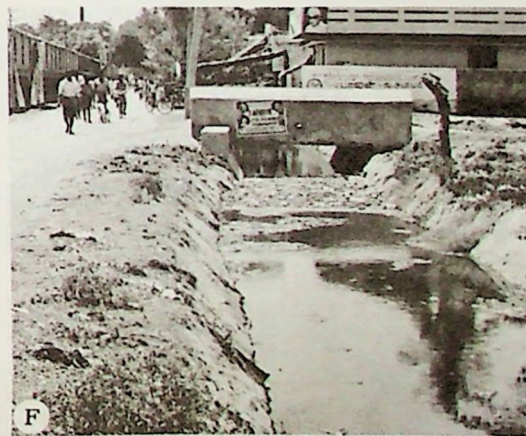
Breeding sites related to water disposal (a) cess pit, (b) box drain, (c) gully trap, (d) blind end drain, (e) cement tank and (f) storm water canal carrying sullage and sewage.
