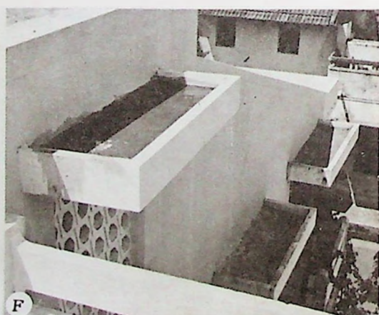
Engineered breeding sites (a) unfinished drain, (b) pillar erected on the storm water canal, (c) electric pole in the drain, (d) curing yard, (e) water stagnates on the roof and (f) sun shade.
